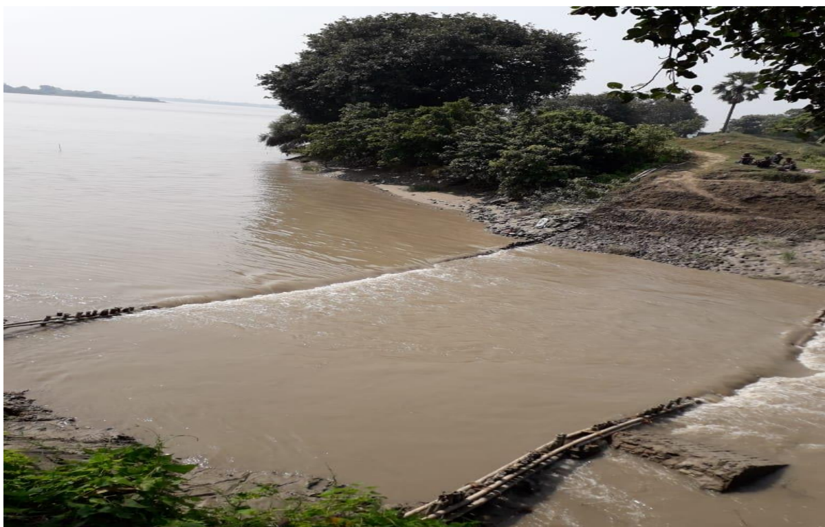
Silt Rich Water Entering Silt-Tanks
